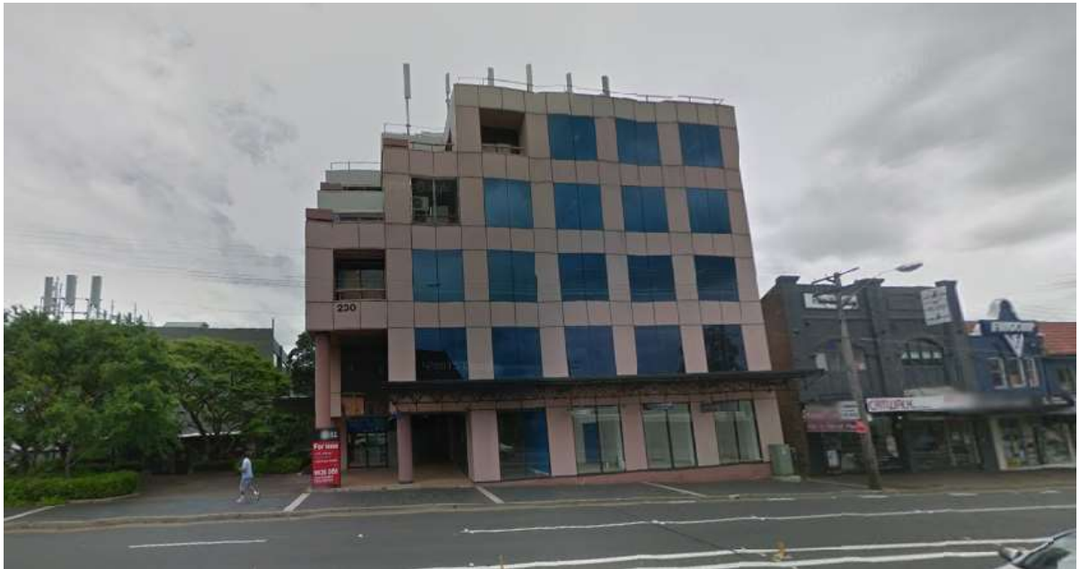
Figure 2: Subject site – View from Victoria Road – existing 5 storey building to be demolished.
